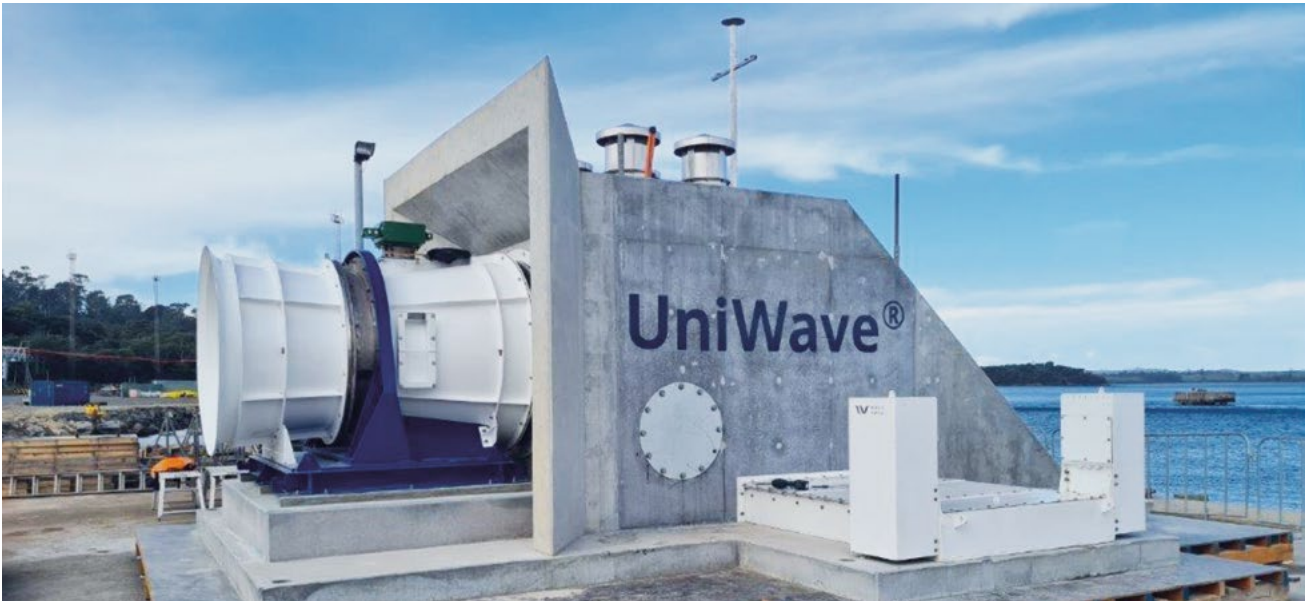
Wave Swell Energy (WSE) prototype under construction (superstructure) to be installed on King Island, Tasmania Courtesy: Wave Swell Energy
